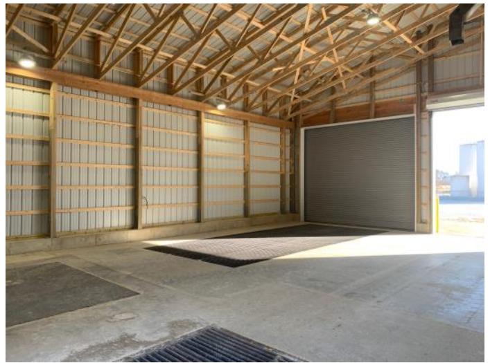
Elma Receiving Pit
